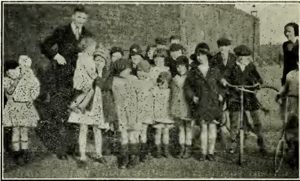
THE BATLEY BRANCH PRIMARY, LEEDS DISTRICT.
